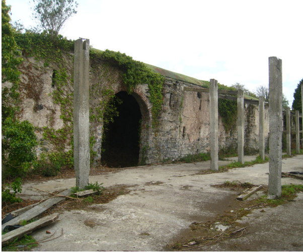
Fig 5: Existing Derelict Historic Coach House Building.
